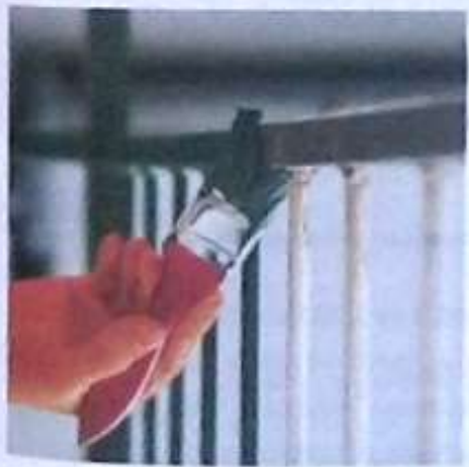
Figure 12.2 Painting prevents rusting
