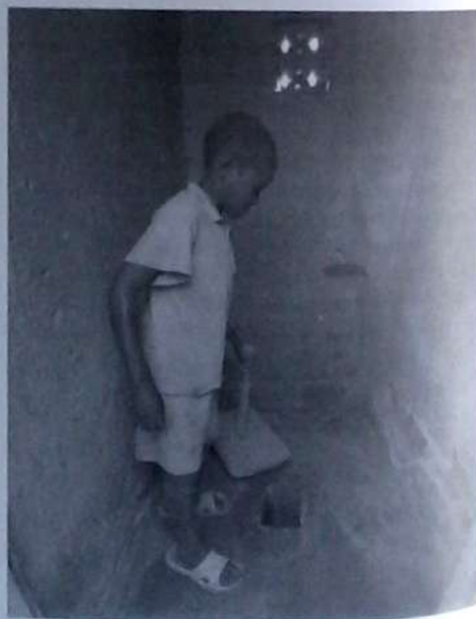
Figure 9.9 a) and b) A diagram of the Blair pit toilet and a picture of it from inside
