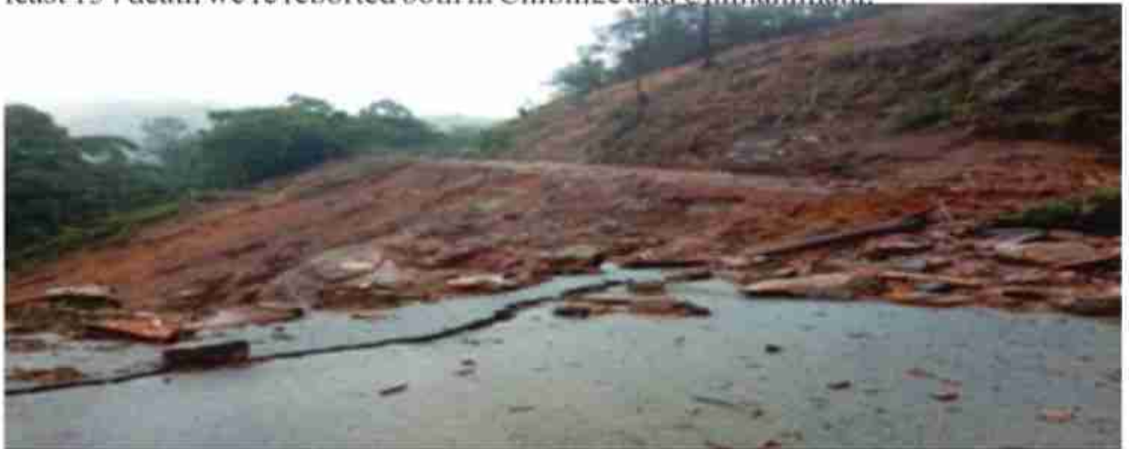
Fig 1.7: Landslides in Chimanimani Picture Courtesy of Stanely Duri
