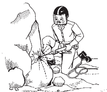
Fig. 6.7 Drilling through bedrock
