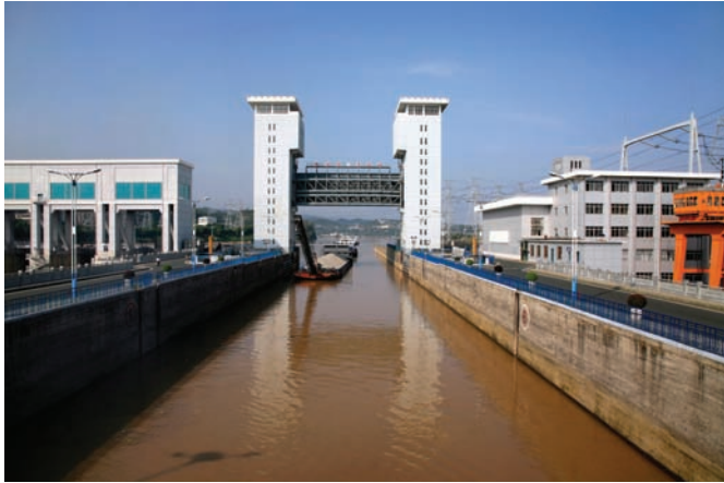
Gezhouba Dam, China – most major projects are evaluated using investment appraisal
