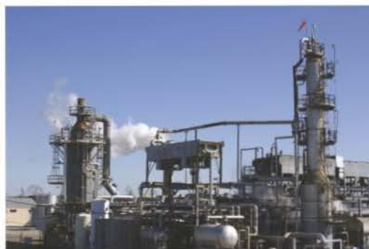
▲ Figure 2 Crude oil is separated into fractions by distillation in cylindrical towers typically 8 m in diameter and 40 m high. Oil refineries vary but a typical one might process 3.5 million tonnes of crude oil per year.
