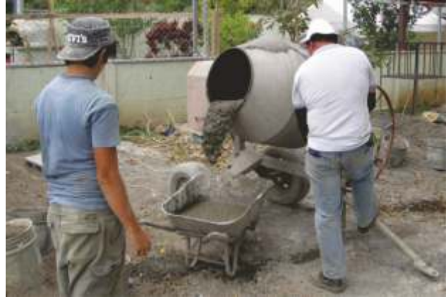
Figure preparing concrete with machine
